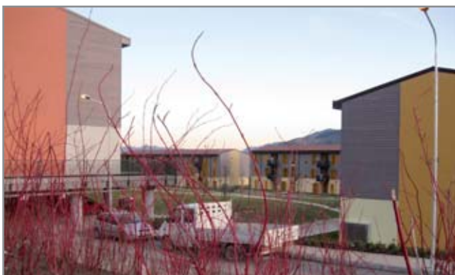
Case ultimate/Construction ends
