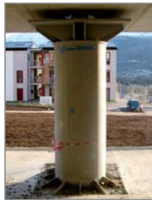
Plinto antisismico sotto la soletta Anti-seismic plinth under the building slab
